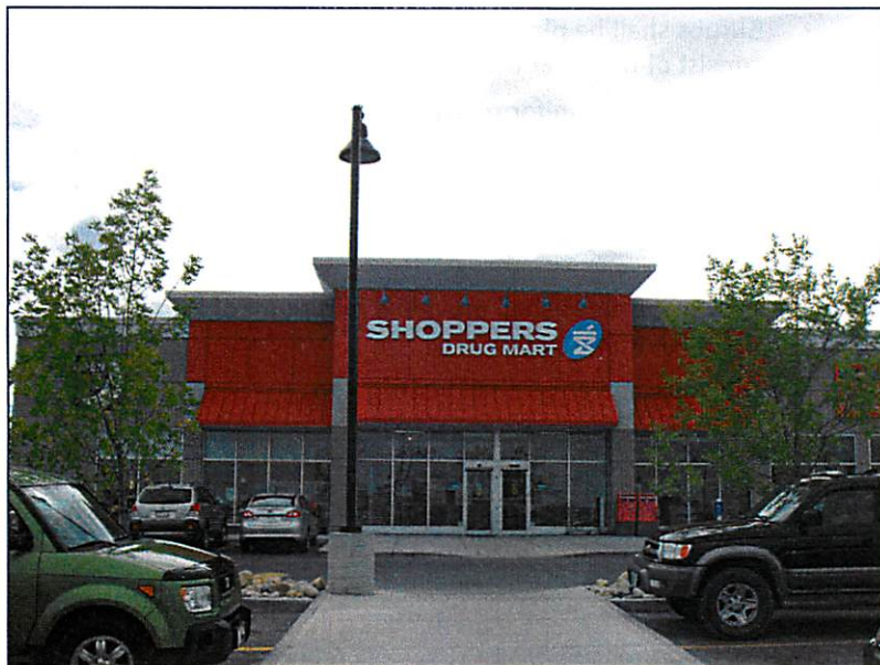
Fig. 62: Parking islands and pick up and drop off areas shall be landscaped.
