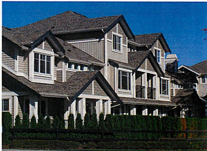
Fig. 15: A variety of roof configurations and details reduce the visual impact of multi-unit residential and blend it more appropriately with the scale and high quality of single-family residential uses.
