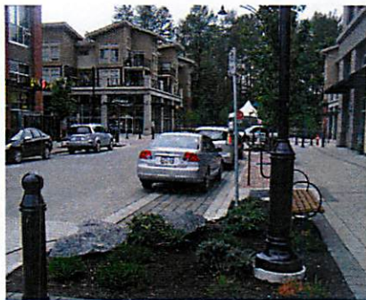
Fig. 19b: Landscape curb extensions along a street or parking lot can be used as a traffic calming device as well as reduce the amount of impervious surface in a development.
