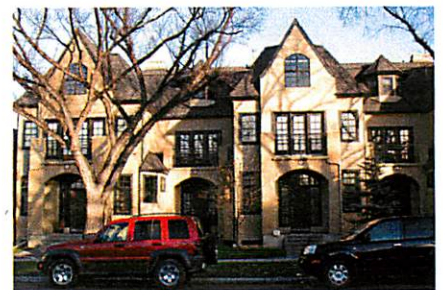
Fig. 14a and b: Well-proportioned, high quality, articulated, multi-family buildings blend into single-family or commercial development patterns.
