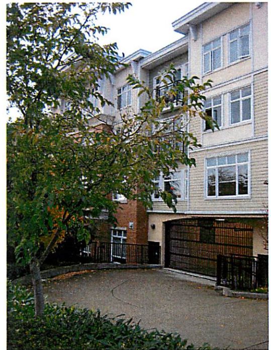
Fig. 20: Underground parkades can be integrated into the building facade so as to be visually appealing from the streetfront.
