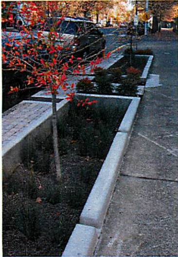
Fig. 19a: Parking design that allows stormwater to enter the planter area as part of a Low Impact Development (LID) stormwater management system can reduce stormwater runoff and recharge local soils with water.
