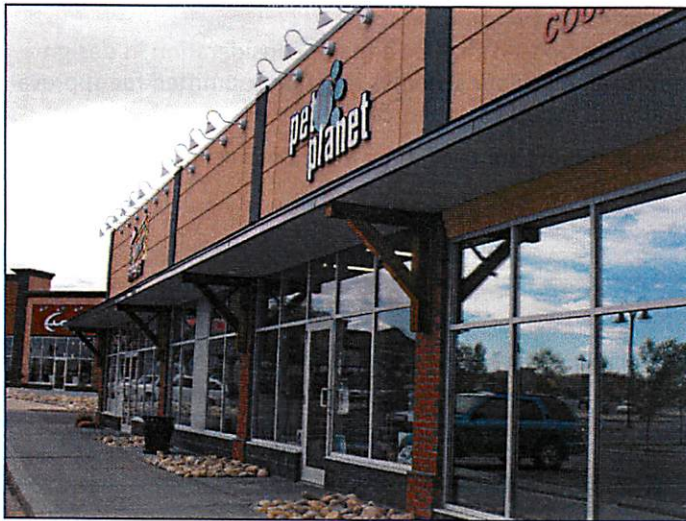
Fig. 68: Goose Neck lighting system in Chestermere's Town Centre provides illumination only where necessary.
